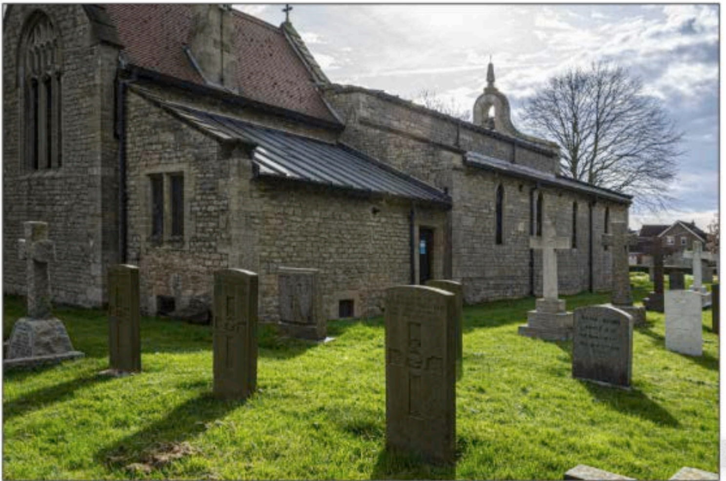
Long and short quoins on the NE corner of the church, and the bellcote at the far (west) end of the nave.
