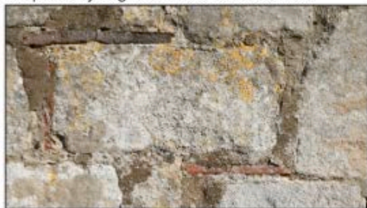
Roman roof tiles used as gap fillers, south wall
